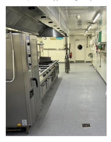
Degafloor's fast curing MMA resin flooring systems are fully cured within just two hours of installation, making them ideally suited to refurbishments where closure periods are limited. Although the hotel had taken the decision to close throughout the installation, it was crucial that the closure was kept to minimum.
